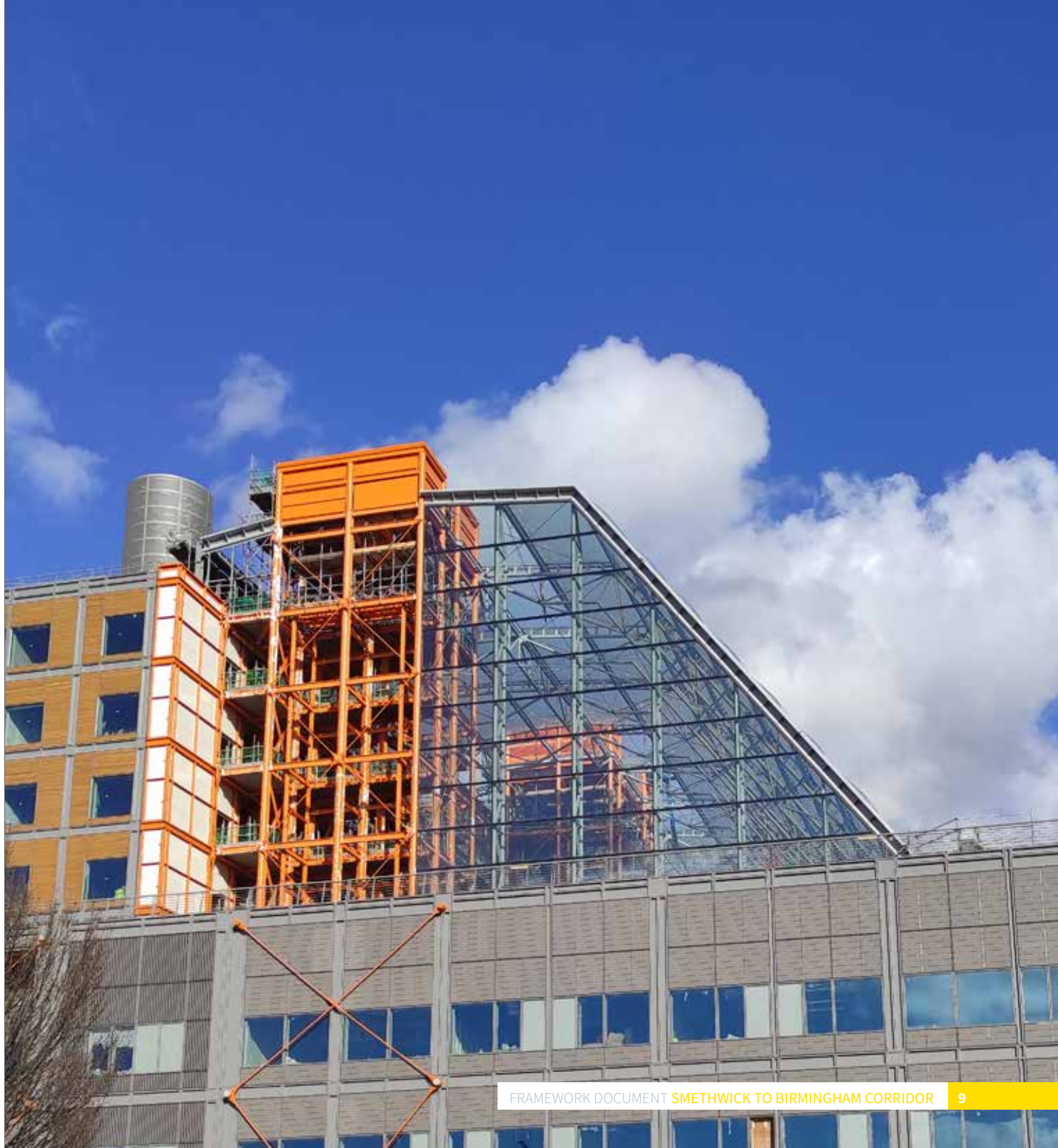
Fig. 1.1 - The new Midland Metropolitan University Hospital (MMUH) is being built at the heart of the Grove Lane area. It is located close to the canal and Moilliett Street Park.
